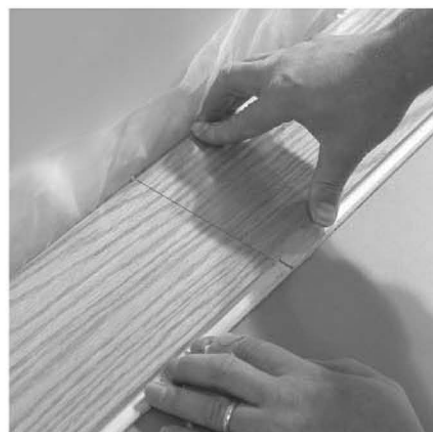
7. Drop second board into place ensuring that the seam is tight.
