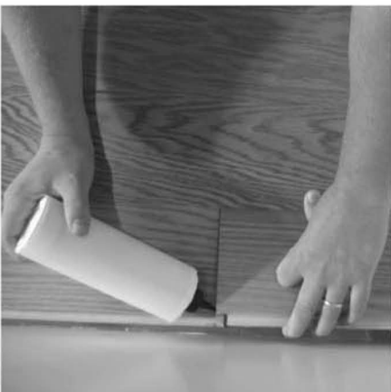
13. Place a bead of glue on the end seams of the last row.
