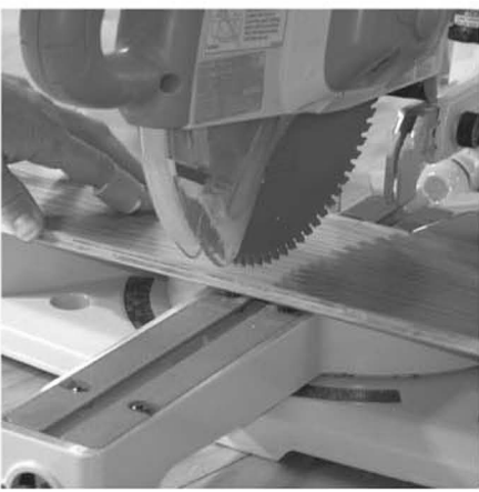
9. The cut board from the first row is used to start the second row.
